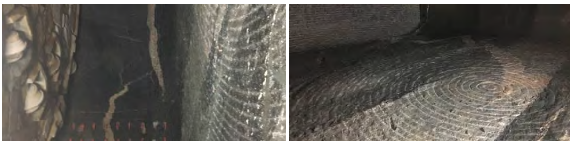
Picture 1 - Tunnel face containing both gneisses and amphibolite
