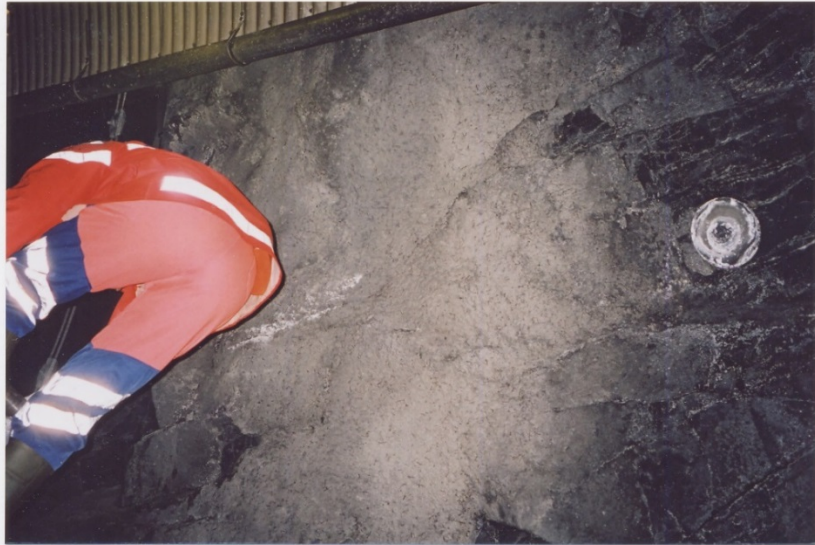
Km 3,132 h.s. God betong.
