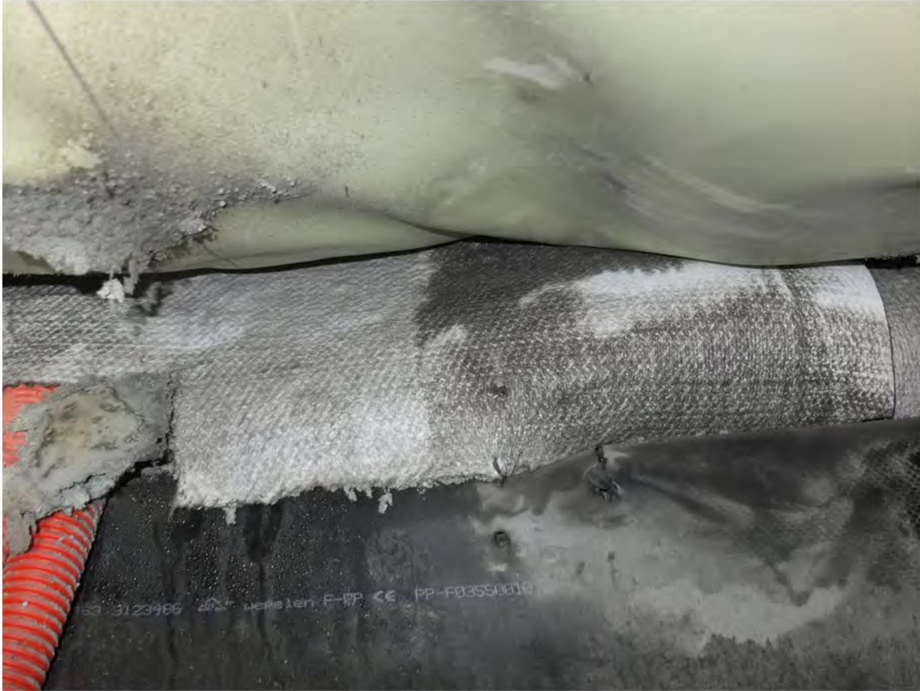
13 Fiberduk under Wapromembran
