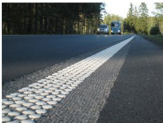
Profilert vegoppmerking nedfrest plant spor
