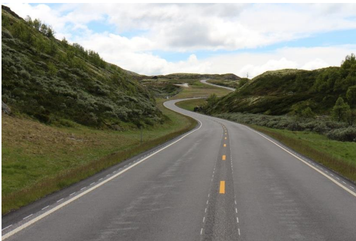
Figur 3.6: Plan midtlinje i plant nedfrest spor (alternativ 3)
