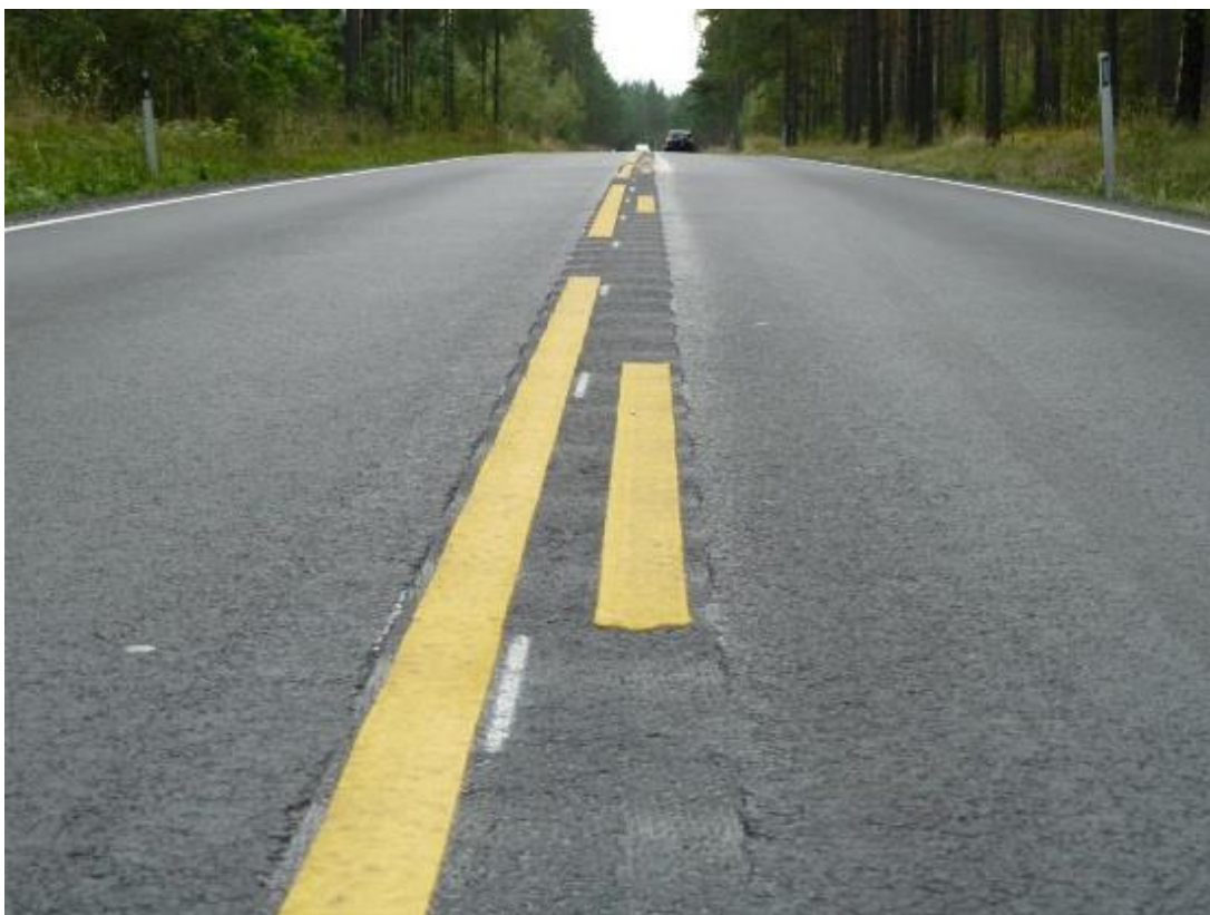
Figur 1.5: Forsterket vegoppmerking i nedfrest sinusrille
