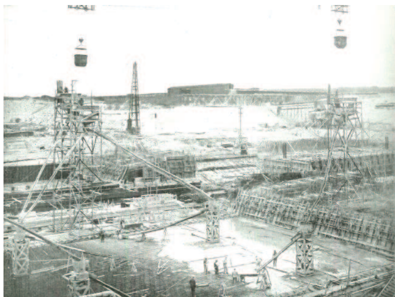
Fig. 1. Construction of the Noordersluis, IJmuiden, including casting of concrete (From Vissers 1927).
