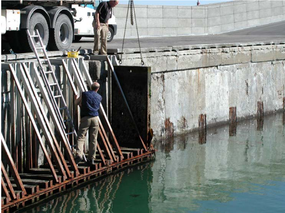
Figure 11 – Aalborg Portland exposure site at Hirtshals harbour. Element being lifted out of rag. Courtesy Dirch Bager 2015
