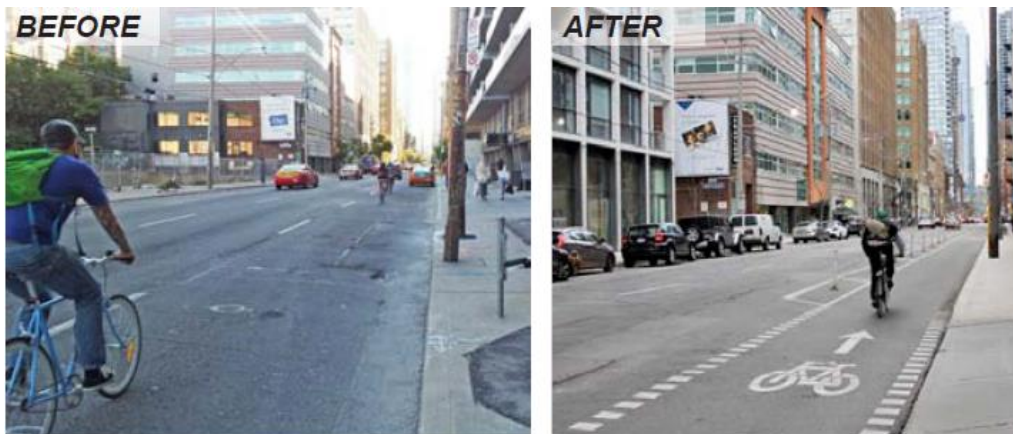
Adelaide Street facing east showing new cycle track.
