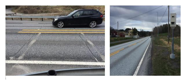
Figure 1 ATK Piezo cables and camera unit
