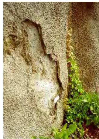
Figure A1-4-2 Left : Overview of sprayed concrete Åkebergveien road cut, city of Oslo in 2000, sitting on Lower Ordovician Alum Shale interbedded with Upper Carboniferous syenite sills (“mænaite”). Cores 1-4 were extracted here. This is the first published case of TSA in Norway (Hagelia and Grønhaug 2000; Hagelia et al. 2001). This steel fibre reinforced wet sprayed concrete was 13 years old and made with SRPC and silica fume. A previous SRPC based 1970 spray was demolished and replaced in 1987. Notice spalling and ferric iron stains, reflecting effects of iron sulfide oxidation. Deformations were also observed. Right : Detail of the spalling (sample “Spall 2) along a 2 cm white mush zone consisting of thaumasite and calcite due to TSA and PCD. Steel fibres were totally destroyed by corrosion in the process. The 1987 spray has not yet been replaced (2010) and is now about 23 years old.
