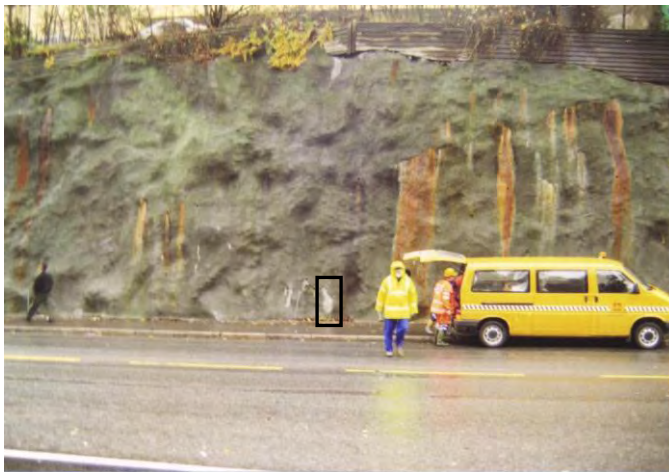
Figure A1-4-2 Left : Overview of sprayed concrete Åkebergveien road cut, city of Oslo in 2000, sitting on Lower Ordovician Alum Shale interbedded with Upper Carboniferous syenite sills (“mænaite”). Cores 1-4 were extracted here. This is the first published case of TSA in Norway (Hagelia and Grønhaug 2000; Hagelia et al. 2001). This steel fibre reinforced wet sprayed concrete was 13 years old and made with SRPC and silica fume. A previous SRPC based 1970 spray was demolished and replaced in 1987. Notice spalling and ferric iron stains, reflecting effects of iron sulfide oxidation. Deformations were also observed. Right : Detail of the spalling (sample “Spall 2) along a 2 cm white mush zone consisting of thaumasite and calcite due to TSA and PCD. Steel fibres were totally destroyed by corrosion in the process. The 1987 spray has not yet been replaced (2010) and is now about 23 years old.
