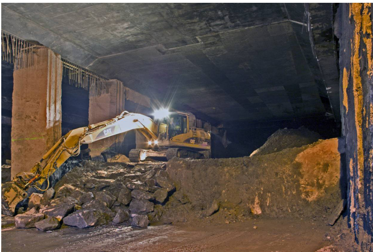
Fig 7.5 – Graving under takplate i gravefloer
