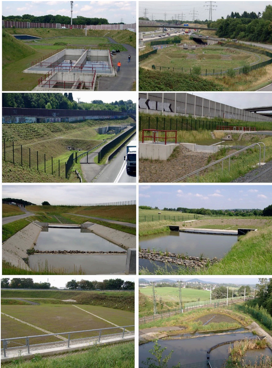
Figure 3.6. Examples of German treatment facilities for highway runoff, showing soil filters as treatment step that follows initial sedimentation and oil separation. Source: Second Bremer Soil Filter-Workshop 26.08.2009, Karl Diefenthal, Landesbetrieb Straßenbau NRW, Regionalniederlassung Rhein-Berg, Außenstelle Köln.
