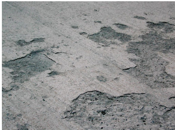
Figure 2.2: Surface scaling
