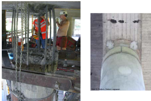
Figure 4.12: Column top cut off and replaced
