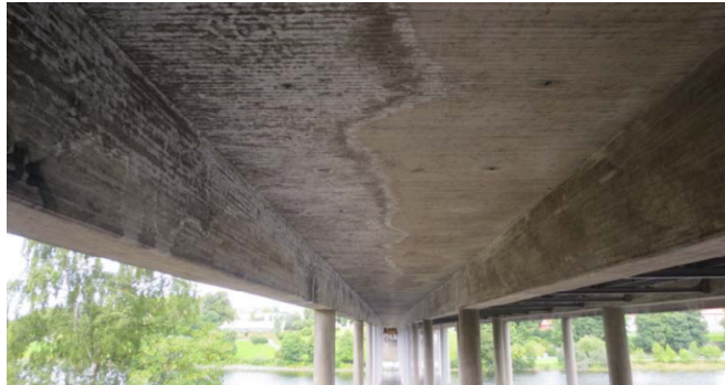
Figure 4.9: Picture taken at axis 1 showing the western side of the bridge deck (Aas Jacobsen, 2013).
