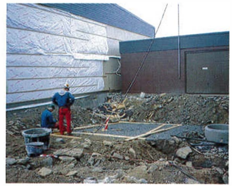
Ny vaskeplass tar form
