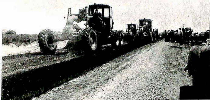
Fig. 10. Road-Mix (Blade-Mixing), Illinois.
