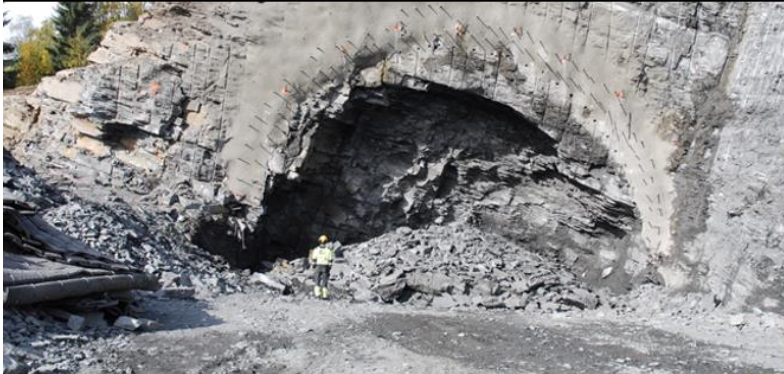
From the first blasting of the Hundorp tunnel
