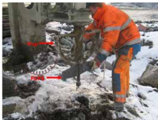
Figur 1-7- 20 FOPS-ving montert under visp for nedpressing (ref. 1)
