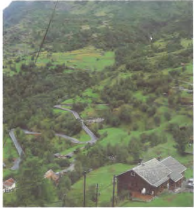
Old roads with a modest standard usually blend well with the landscape, but capacity and safety create problems. Geiranger. Photo: Mari-Lise Sjong
