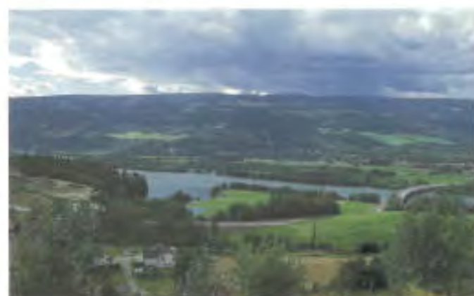
At Jorekstad in Oppland, a new link between the E 6 and Rv 255 avoided the Lågen Delta Nature Reserve. Thickets along the river separate the new road from the reserve, protecting it. This alignment, however, cost more cultivated land. The bridge over the River Lågen was extended to reduce disturbance to an abandoned river bed and give better conditions for people walking beside the river. Photo: Kari Øvrelid
