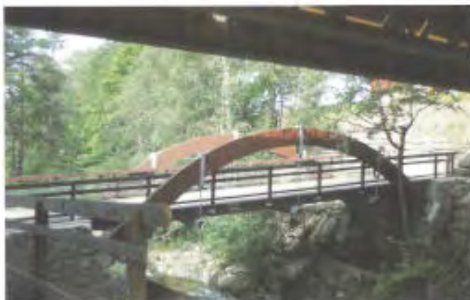
As part of the Mesnadal project in Lillehammer, footbridges, underpasses and well-planned paths were constructed to the continuous system of green spaces as intact as possible. Photo: Kari Øvrelid
