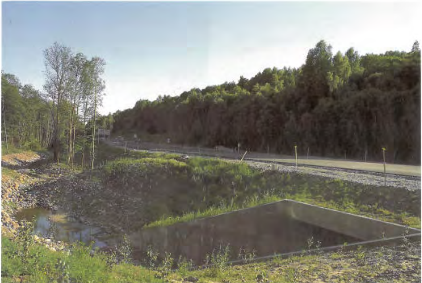
Near Vinterbru in Ås, Akershus, the original proposal for a new stretch of the E 6 involved culverting Årungselva for 200 metres. This would have been a serious detriment to a valuable stream containing both sea trout and salmon. The stream was instead re-routed in a new bed alongside the road, specifically designed to create good conditions for fish to grow up in. (NB: the stream had dried up when this picture was taken.) A short culvert under the road was constructed with thresholds
