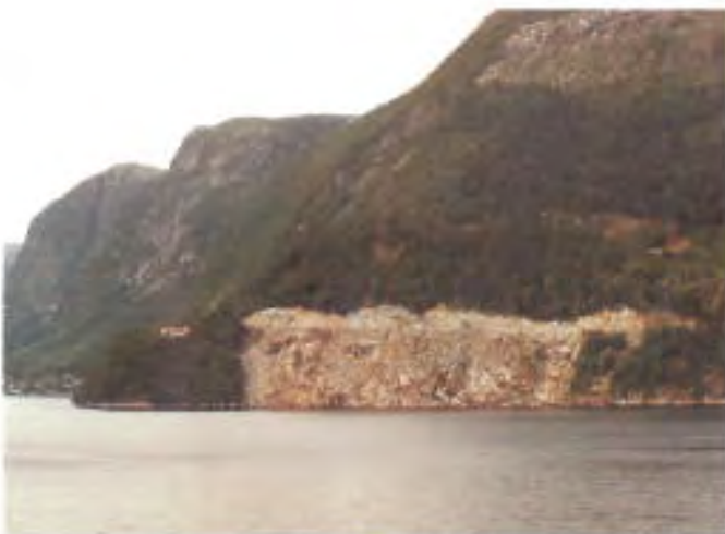
Because heavy mechanical equipment is used, large eyesores are frequently created when roads are built or widened in difficult terrain. Cheap ways of moving rock and earth make it more economical to construct large cuttings and embankments than smaller ones limited by walls. Vadheim, Sogn & Fjordane. Photo: Anon.
