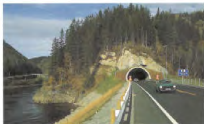
At Støren in Sør-Trøndelag, the E 6 was routed through a tunnel to avoid destroying a crag which is an important element in the landscape. The rest of the shore zone was destroyed. Photo: Egil Lundebrekke
