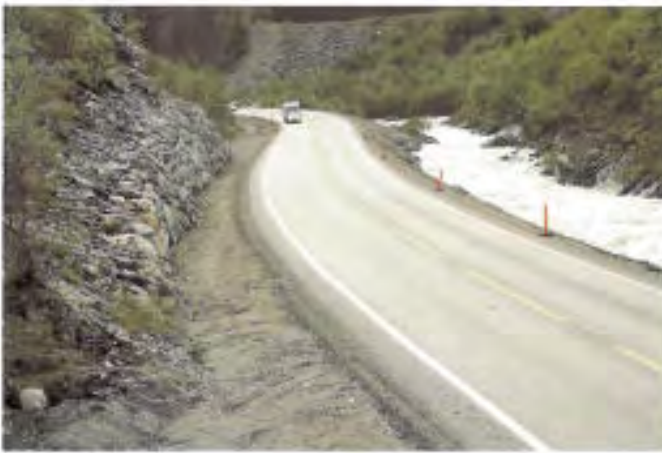
It can be difficult accommodating a high-standard road to a narrow valley floor. The impression of a fine wall is spoiled by a destroyed shore zone. E 6 in Drivdalen, Sør-Trøndelag. Photo: Sunniva Schjetne
