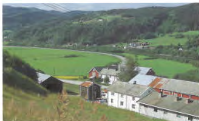
At Horg in Sør-Trøndelag, a new stretch of the E 6 was placed close to fit into the river. The road only slightly disturbing the landscape, thus protecting the shore zone and the rich diversity of species in the undergrowth along the river. Photo: Kari Øvrelid
