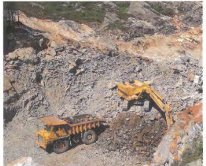
Blasting technique, Askøybroen in Hordaland. Photo: Erling Grønsdal
