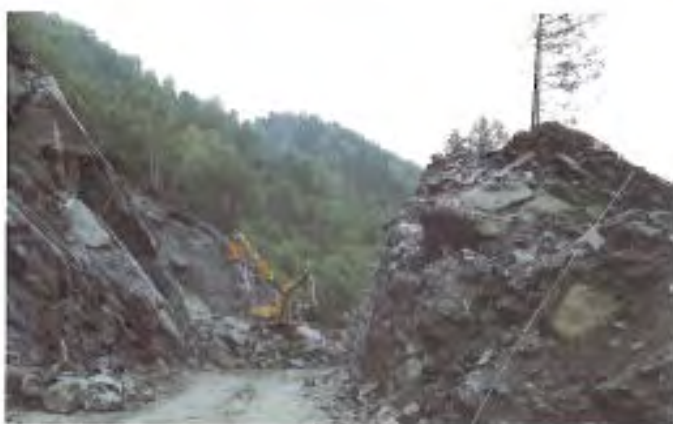
Removing rock and earth, Hordaland. Photo: Erling Grønsdal
