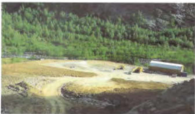
Site where superfluous stone and earth is dumped and equipment and stores are kept, Samnanger, Hordaland.
