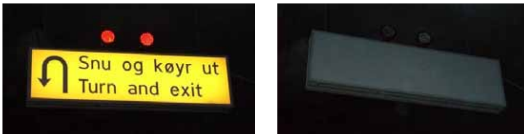
Figure 2.10 Two-position sign in active and passive positions.
