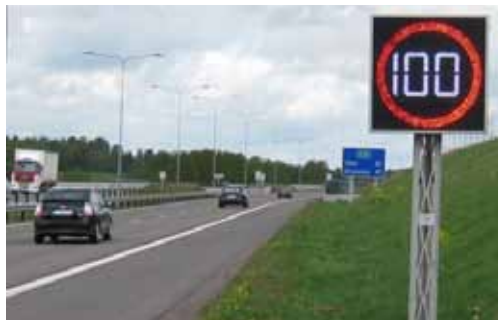
Figure 2.2: Example of a light-emitting up matrix sign.
