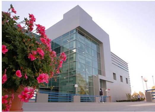
Figur 1: Regional Transportation Management Center.
