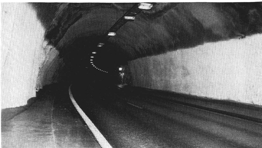
Fig 4 PE foam lining fire protected by lightweight shotcrete
