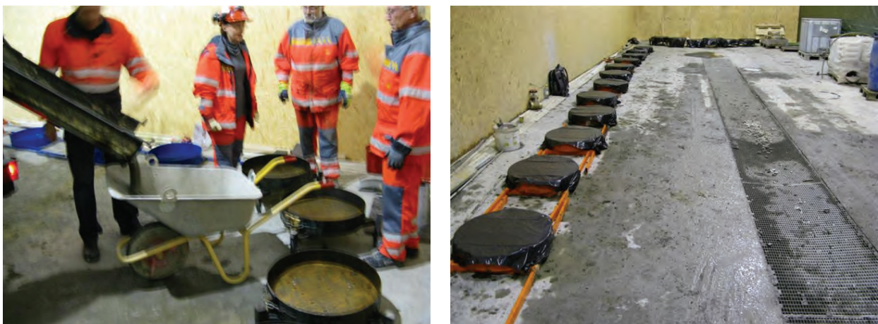
Fig. 4.2 Arrival of the concrete truck and loading of concrete (left). The 18 panels after end of casting and covering with plastic foil (right)
