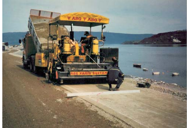
Figure 6: Casting roller-compacted concrete on one of the first projects.
