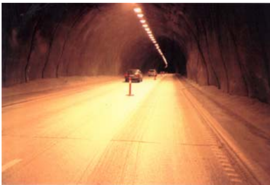
Figure 14: Picture from a tunnel with face/stud – milling work. There are very little experiences with this method in Norway.
