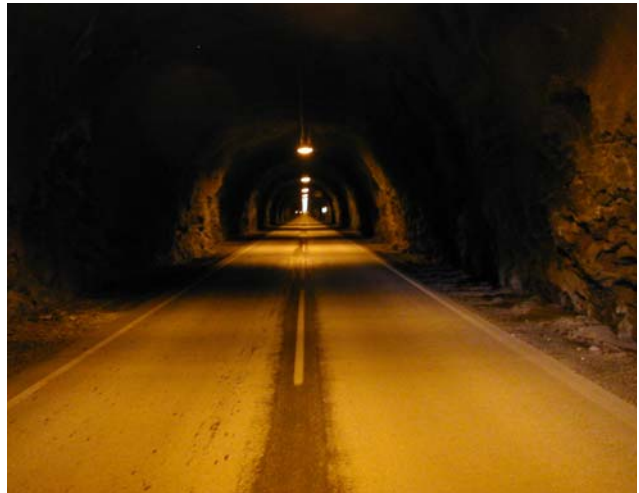
Figure 2: The picture shows a roller-compacted concrete pavement in Steigen Tunnel.
