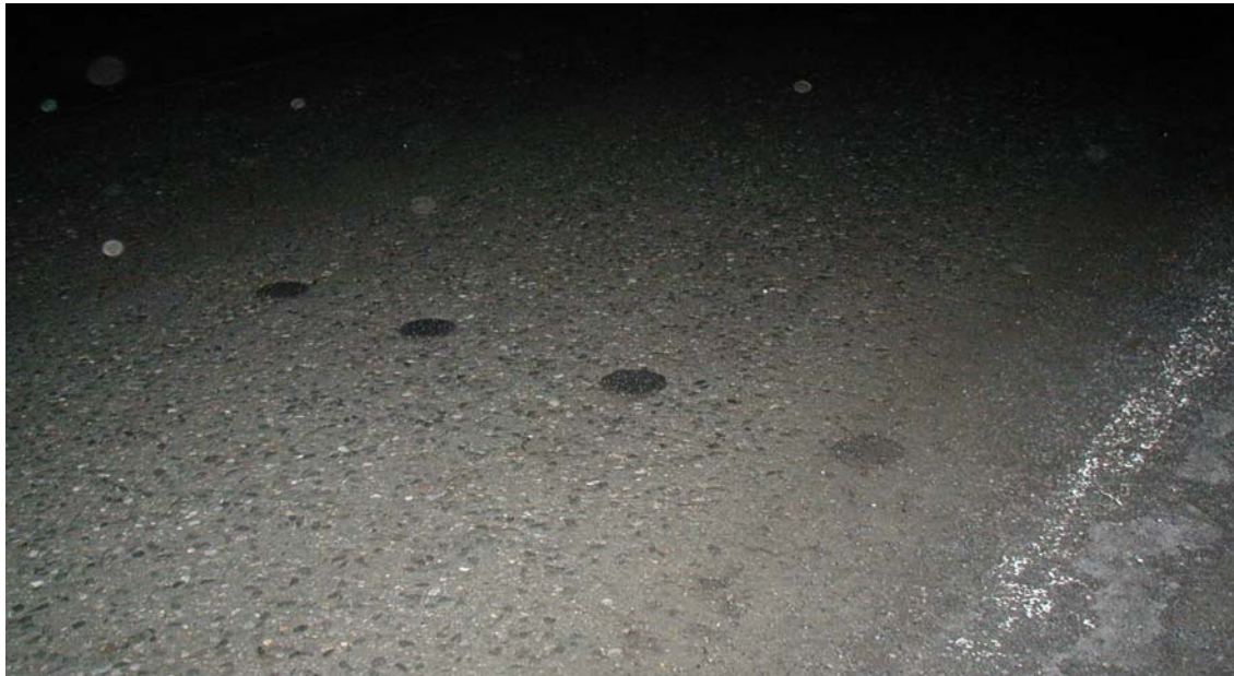
Figure 13: Concrete surface with test cores.
