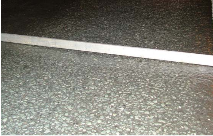
Figure 12: Example of good distribution of aggregates on the surface.
