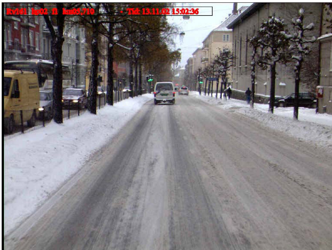
Figur V1.14: Rv 161: Rv 161, ny asfalt
