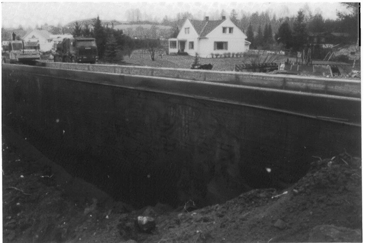
Figure 7. Shot-crete spraying in progress.
