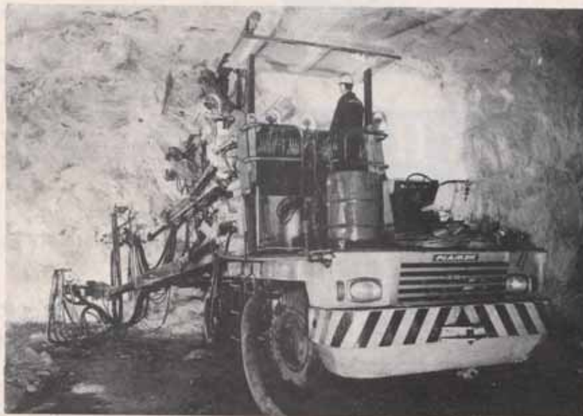
Borerigg for tunnel- boring, 4 bommer + dekurs. Atlas Copco boreutstyr, norskbygget understell
