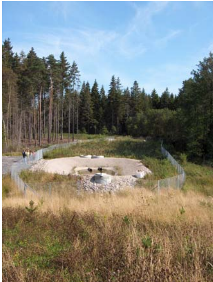
Figure 12: Stormwater pond at E6 in Råde (Norway) which consists of a separate sedimentary basin with hard bottom followed by a shallow wetland filter (0.5 m) with overflow to the stream (Photo: Roger Roseth).
