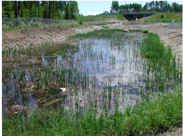
Figure 12: Stormwater pond at E6 in Råde (Norway) which consists of a separate sedimentary basin with hard bottom followed by a shallow wetland filter (0.5 m) with overflow to the stream (Photo: Roger Roseth).
