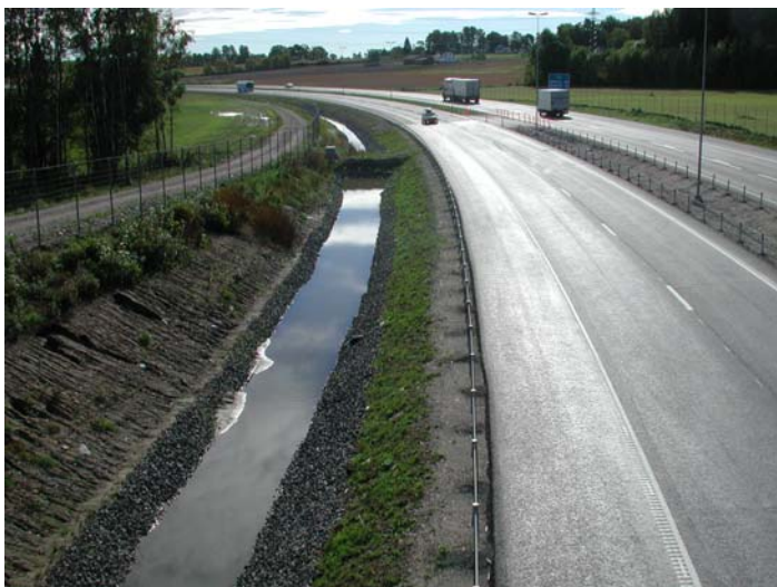
Figure 13: Water-filled gully with local thresholds/dams for infiltration and sedimentation of the added surface water.
