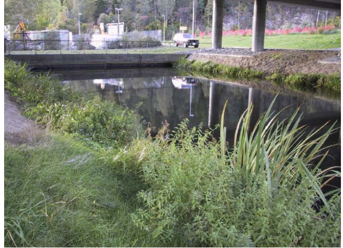
Figure 11: Stormwater pond at E6 Skullerud in Oslo (Norway) with an integral and closed soakaway and water depth of 1.5 m (From Åstebøl and Coward 2005).
