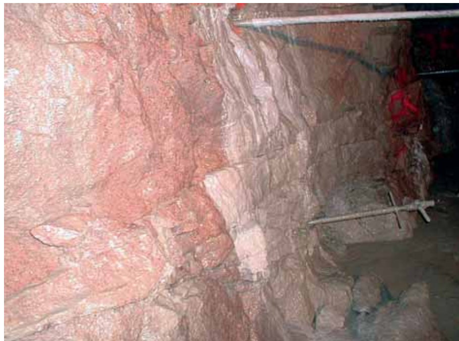
Figure 16 Grouting in the Hagan tunnel syenite
