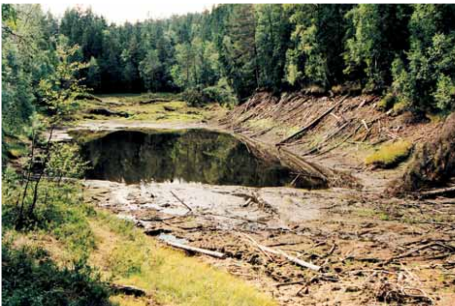
Figure 10 The tarn Puttjern which is situated above the Romeriksporten tunnel. It was nearly drained due to tunnel leakages, and later, due to response from neighbours, restored with grouting and permanent water infiltration (Photo: L. Erikstad).
