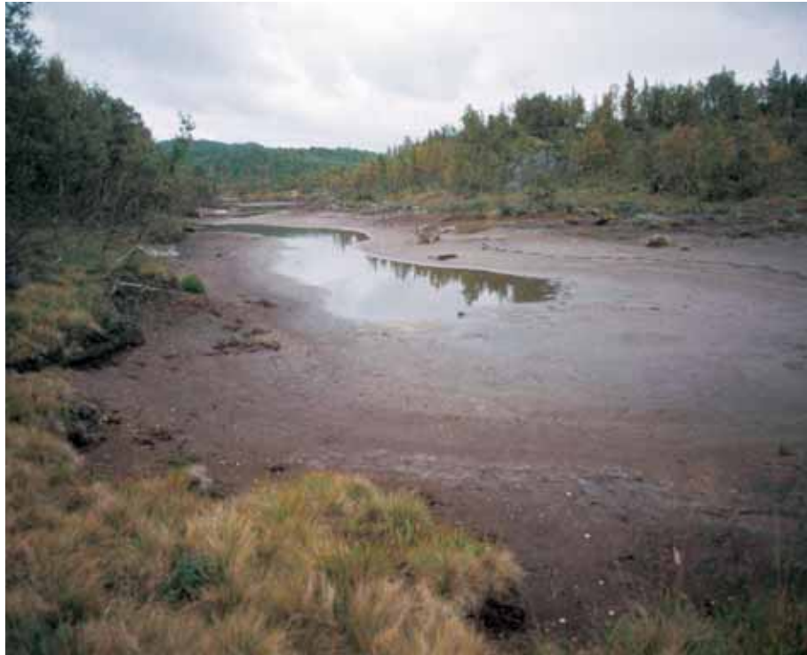
Figure 12 Partly drained lake above the Tokke hydropower tunnel. Seasonal leakages cause significant variations in the water level. (Photo: A. Often).
