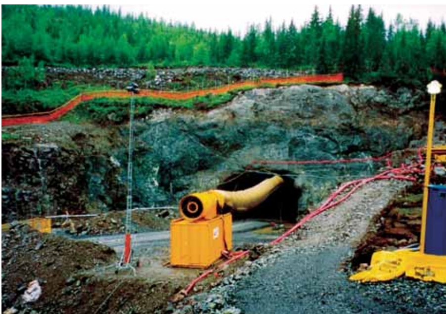
Figure 1 The Lunner tunnel, built at Rv 35 north of Oslo.
