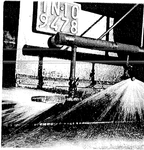
Figure 8. K40 and P40100 nozzles on sprinkling bar.
