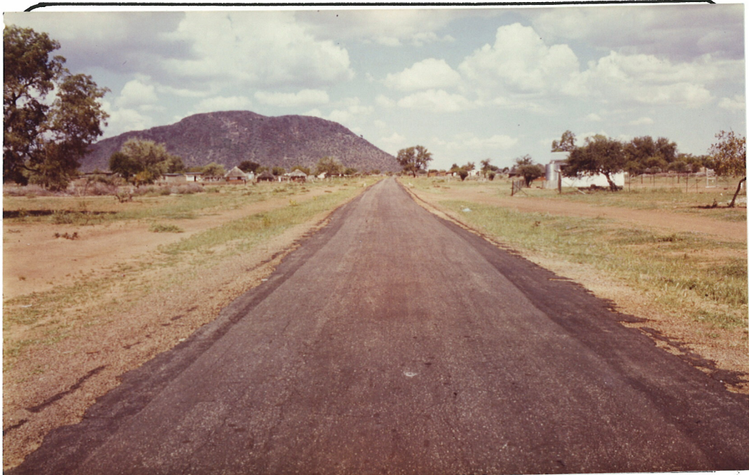
General view, section seen from km.17.5...to km.18.5...
