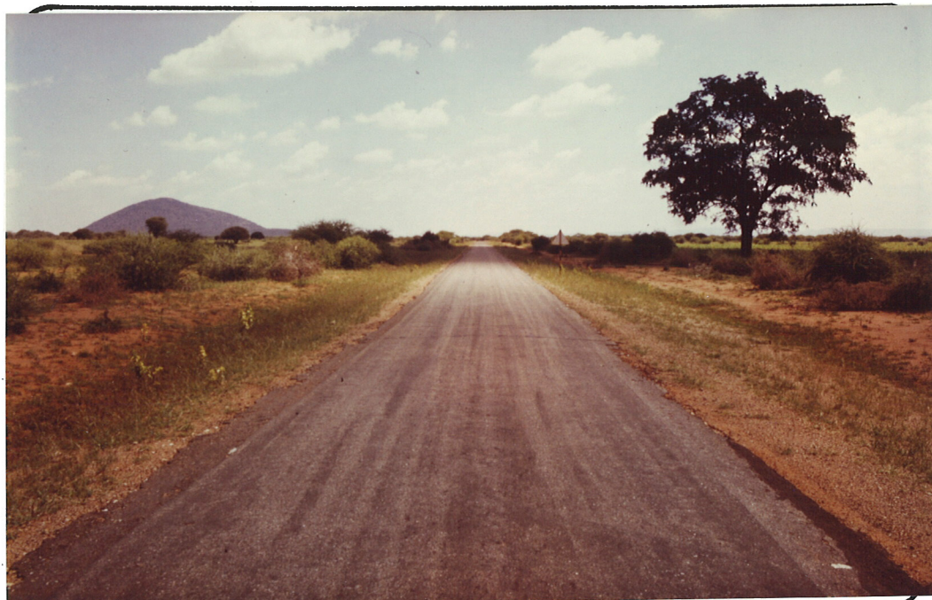
General view, section seen from km. 11.235.....to km. 11.0.....
