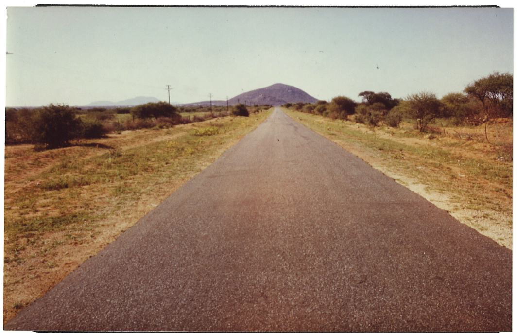
General view, section seen from km. 1.5... to km. 2.5...
