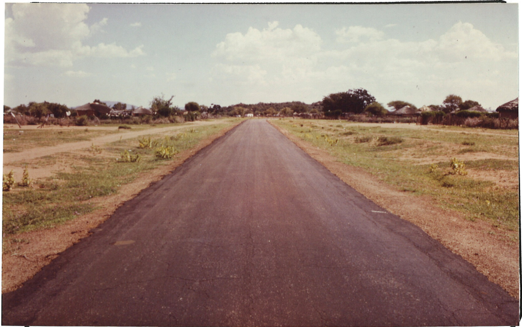
General view, section seen from km.18.5...to km.17.5...
