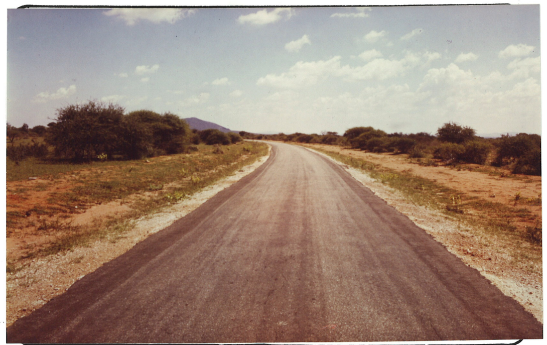
General view, section seen from km. 13.0.....to km. 12.0.....
