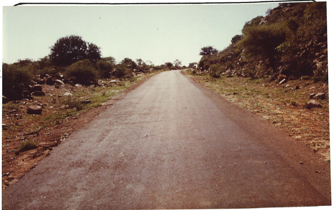
General view, section seen from km. 5.7... to km. 6.7...
