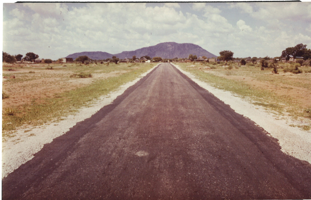
General view, section seen from km. 15.5... to km. 16.5...
