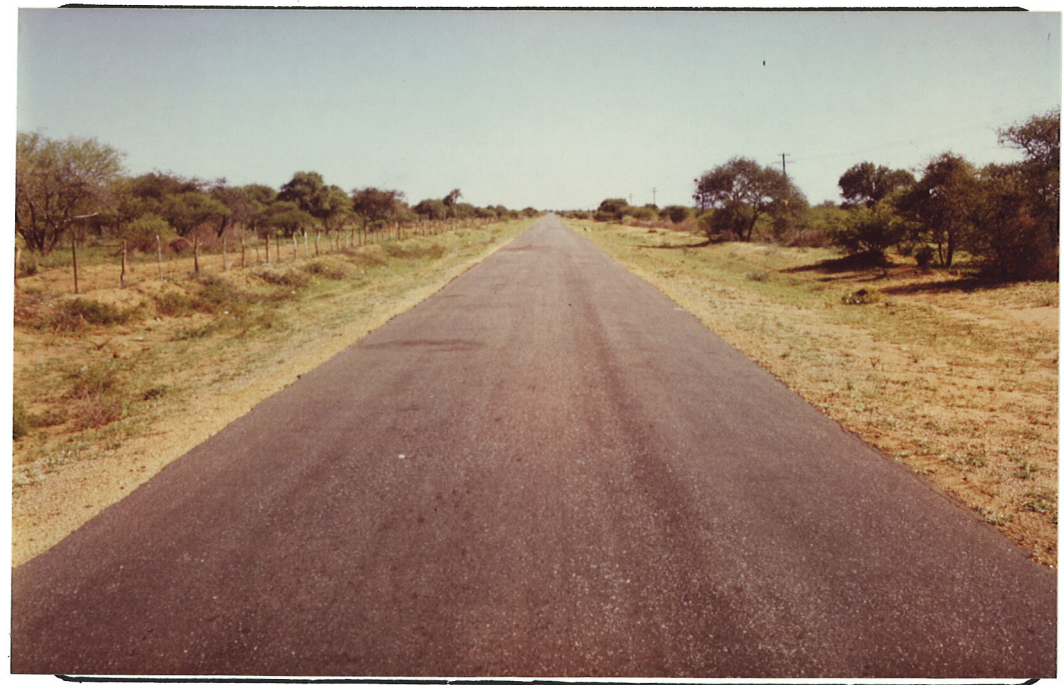
General view, section seen from km. 2.5... to km. 1.5...
