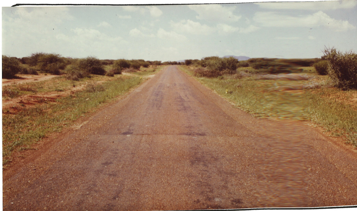
General view, section seen from km. 10.0 to km. 11.0
