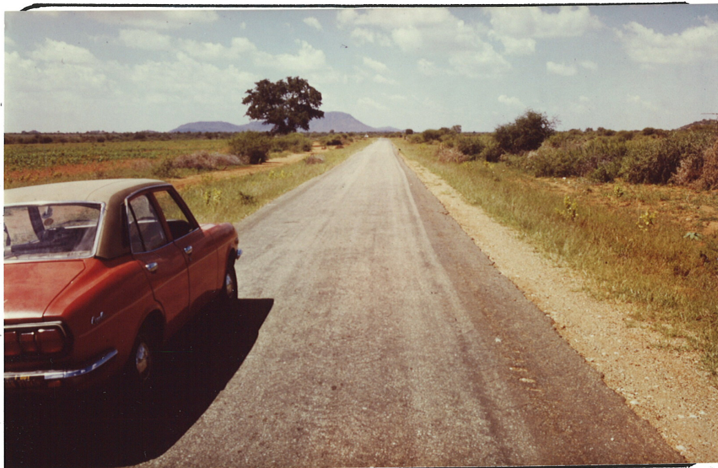
General view, section seen from km. 11.0.....to km. 11.235
