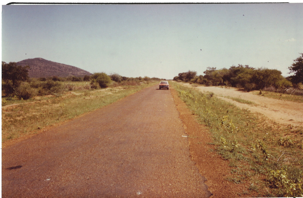
General view, section seen from km. 9.0... to km. 8.0...
