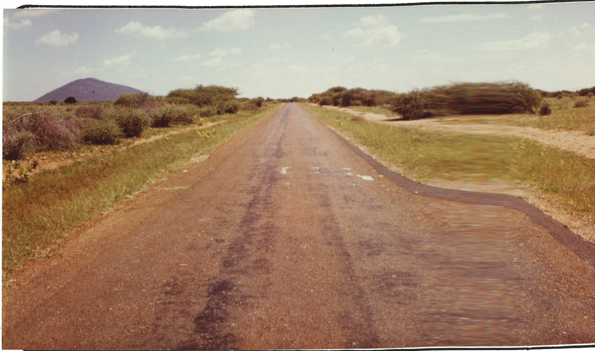
General view, section seen from km. 11.0 to km. 12.0
