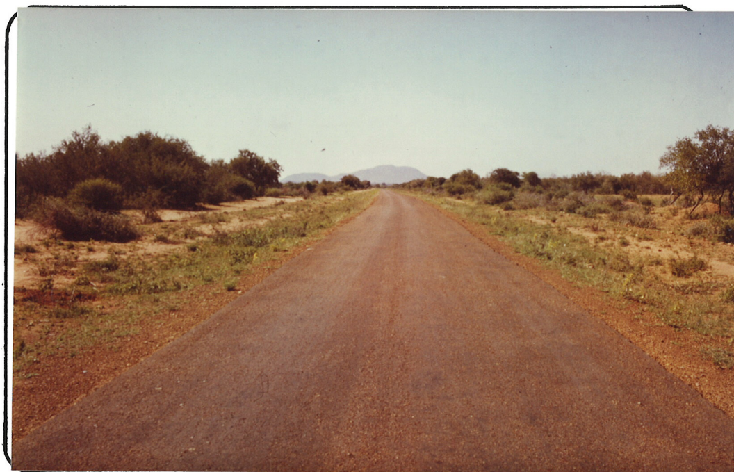
General view, section seen from km. 8.0... to km. 9.0...
