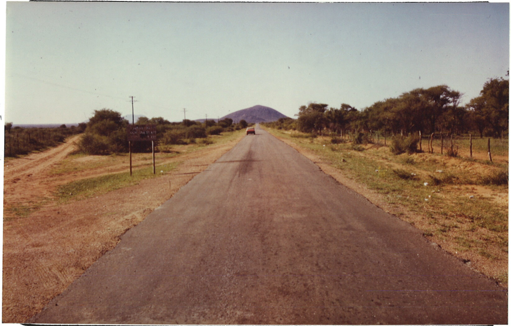
General view, section seen from km. 0.1.....to km. 1.1.....
