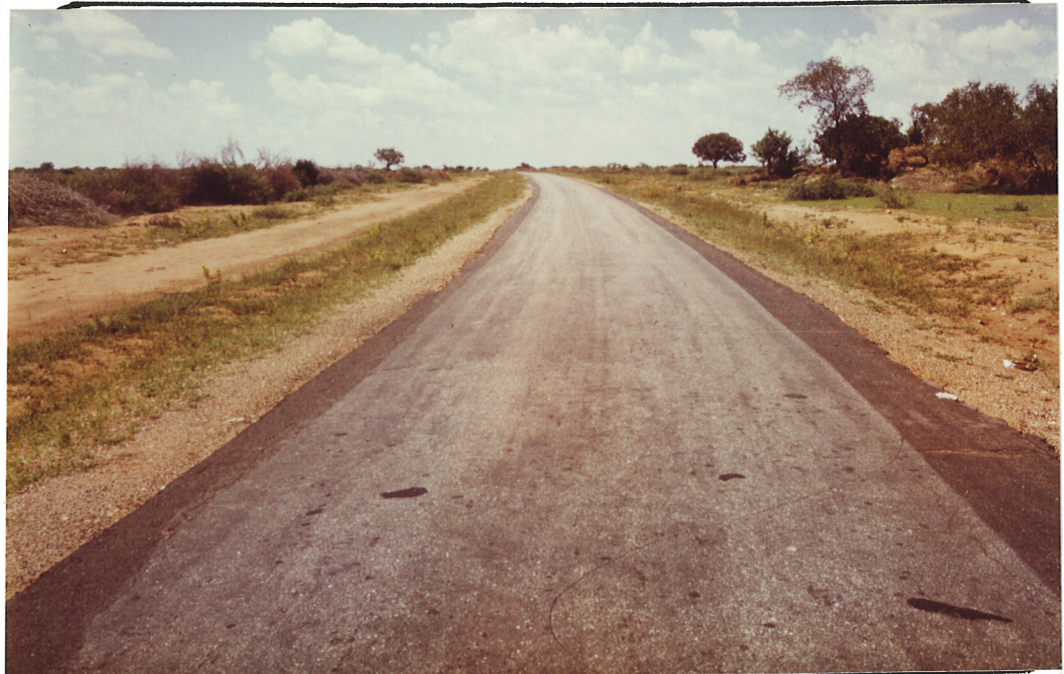
General view, section seen from km. 12.0.....to km. 13.0.....
