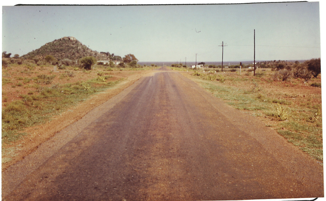
General view, section seen from km. 6.7... to km. 5.7...
