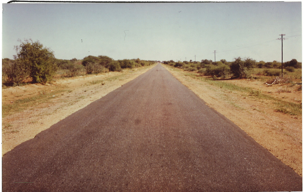
General view, section seen from km. 1.1.....to km. 0.1.....
