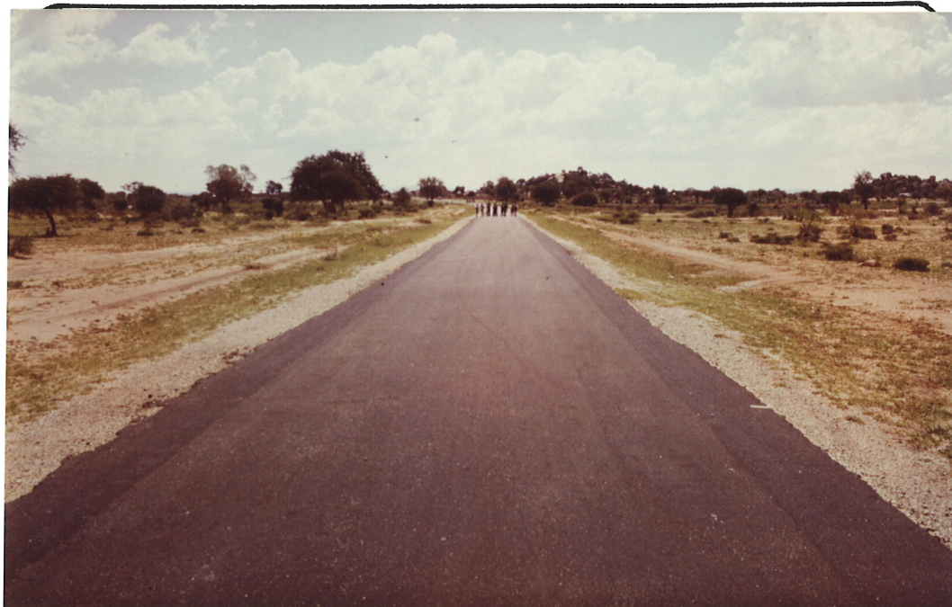
General view, section seen from km. 16.5... to km. 15.5...
