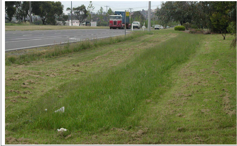
Figure 1. Grass swale, Melbourne 2004
