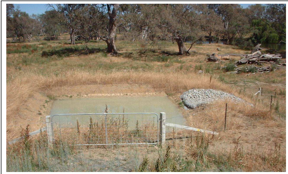
Figure 4. Sedimentation Pond on Calder Freeway, Victoria 2004
