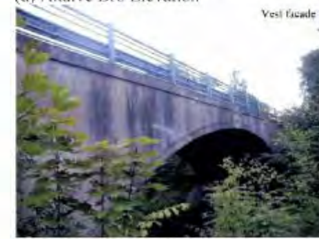
(f) Avdebo Arch Bridge
