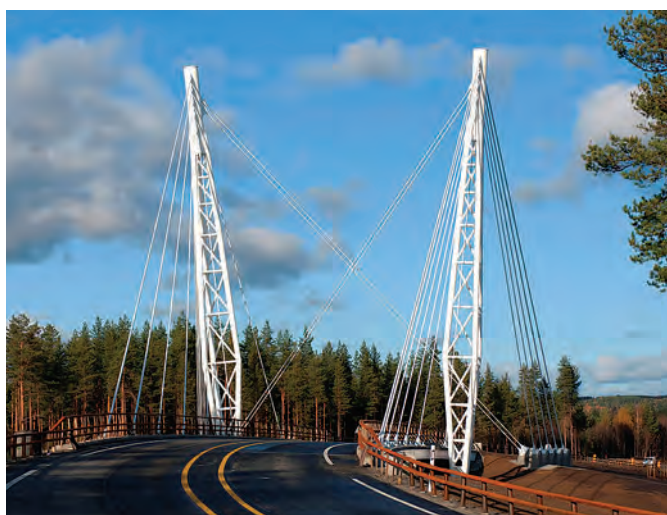
Fig. 8. The towers seen from the bridge
