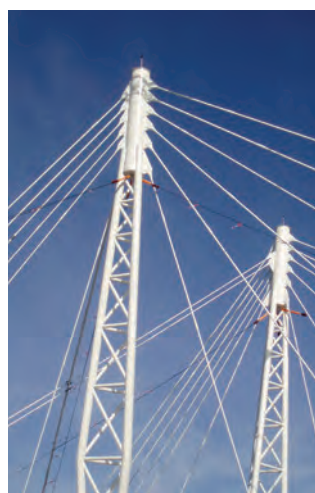
Fig. 10. The towers and the cables
