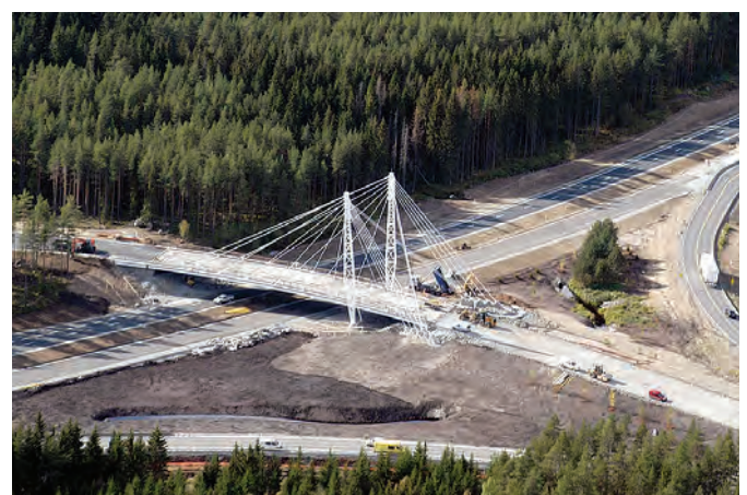
Fig. 15. Photo from the air of the bridge and the road
