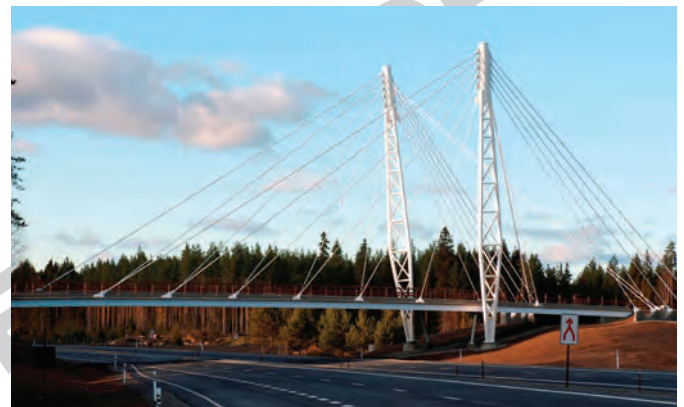
Fig. 2. The bridge seen from south
