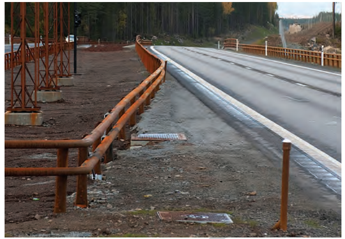
Fig. 3. The road with guard rails in cor-ten steel
