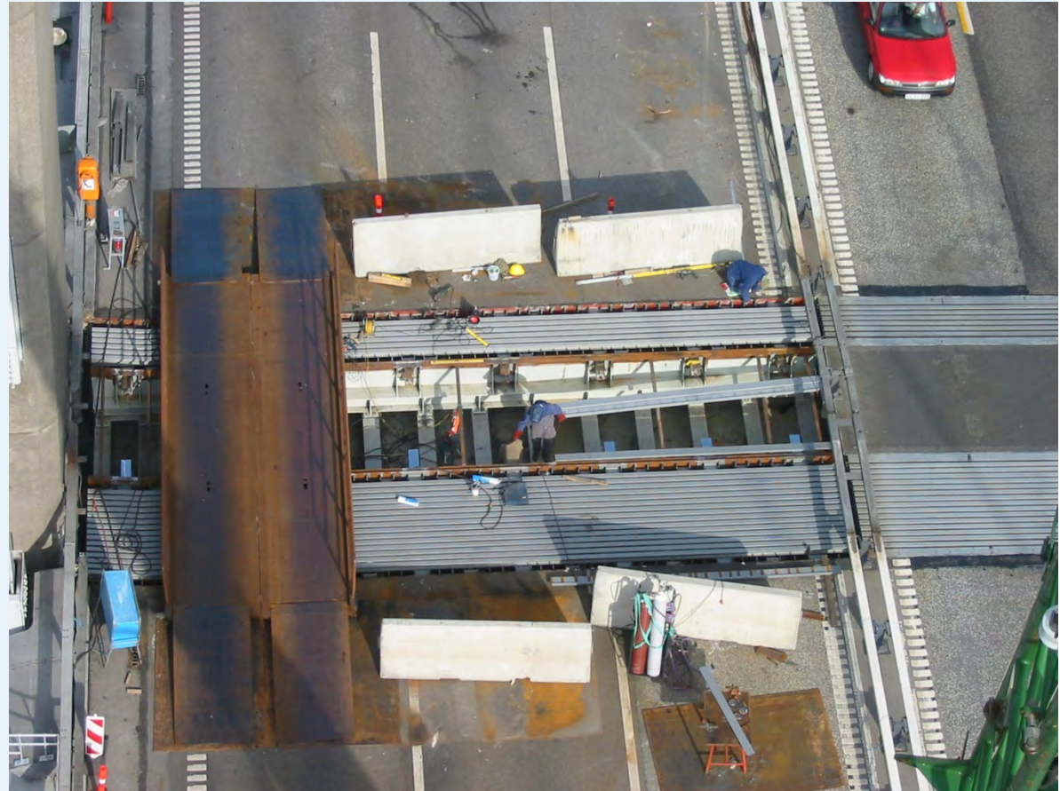
Little Belt Bridge, Denmark
