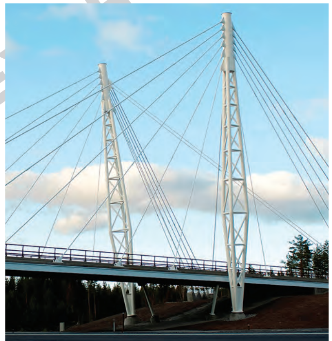
Fig. 14. The towers seen from the road guardrails
