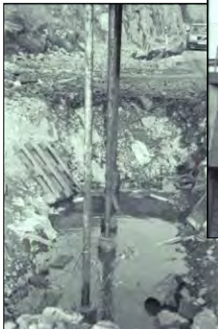
Steel stays anchorage in the bedrock
