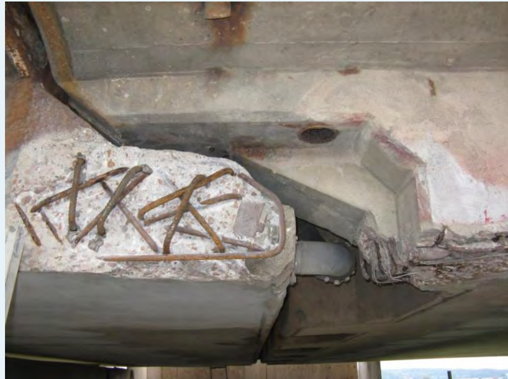
Svendborgsund Bridge, Denmark
