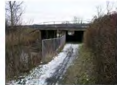
(b) Bridge at Norreso Elevation
