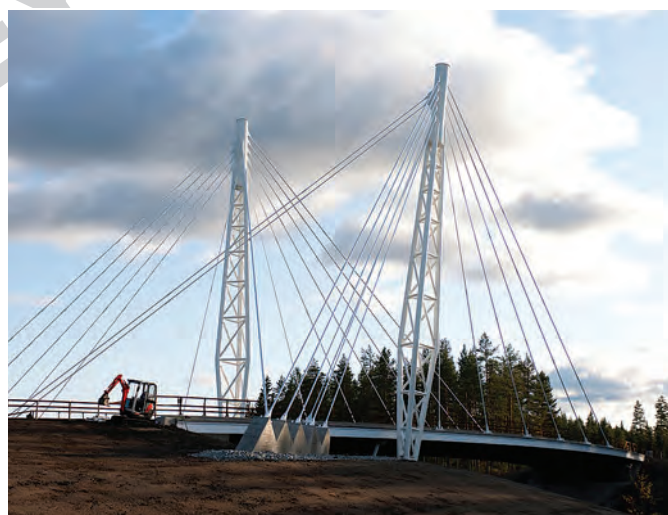
Fig. 9. The towers seen from a sideroad
