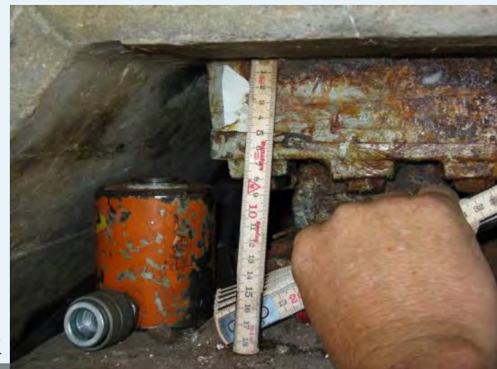
Svendborgsund Bridge, Denmark
