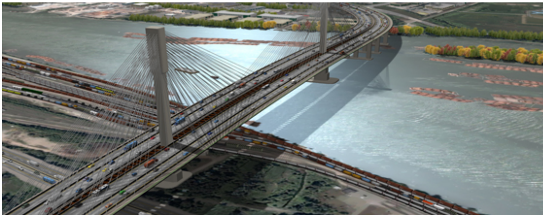
New Port Man Bridge – verdens bredeste, 10 kjørebaner.
