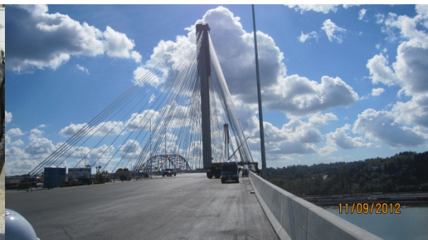
New Port Mann Bridge.
