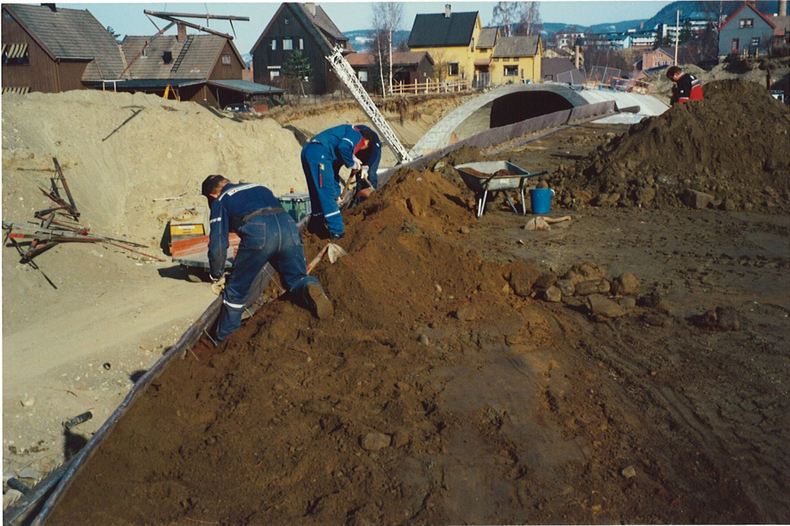
Fig. 5 Fine grained vegetation soil including seed in the front (0,5 m thick)
