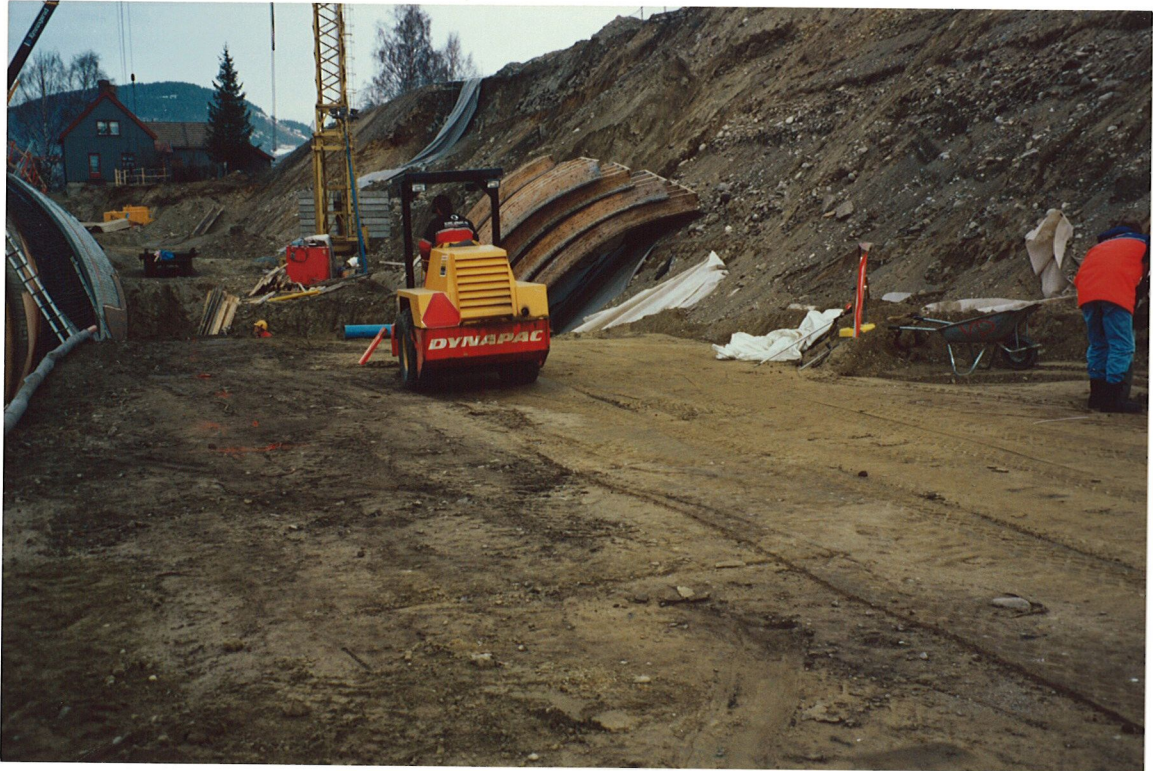
Fig. 3 Compaction of the silty, sandy gravel
