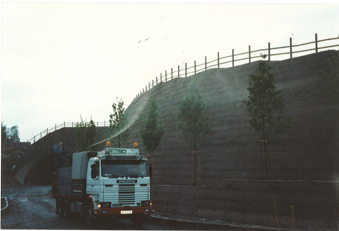
Fig. 8 Hydroseeding the slope
