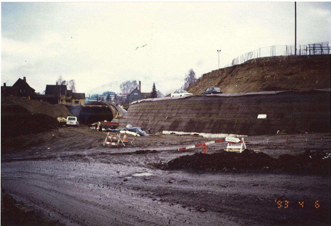
Fig. 4 Construction of the 11. lift
