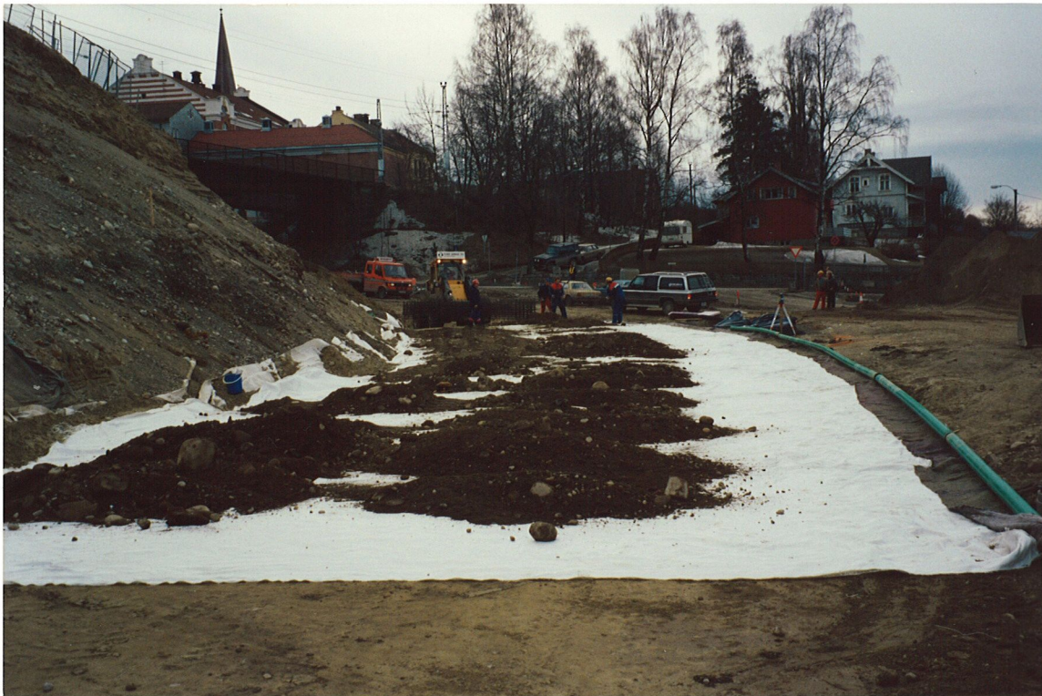
Fig. 1 Drainage layer of gravel before construction
