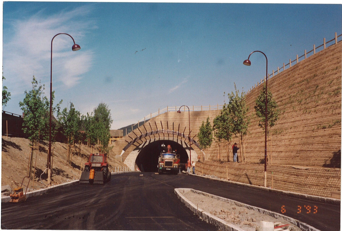
Fig. 10 Finished slope and asphaltting the road
