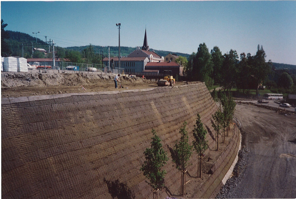
Fig. 7 Inclinator installation on top of the reinforced slope
