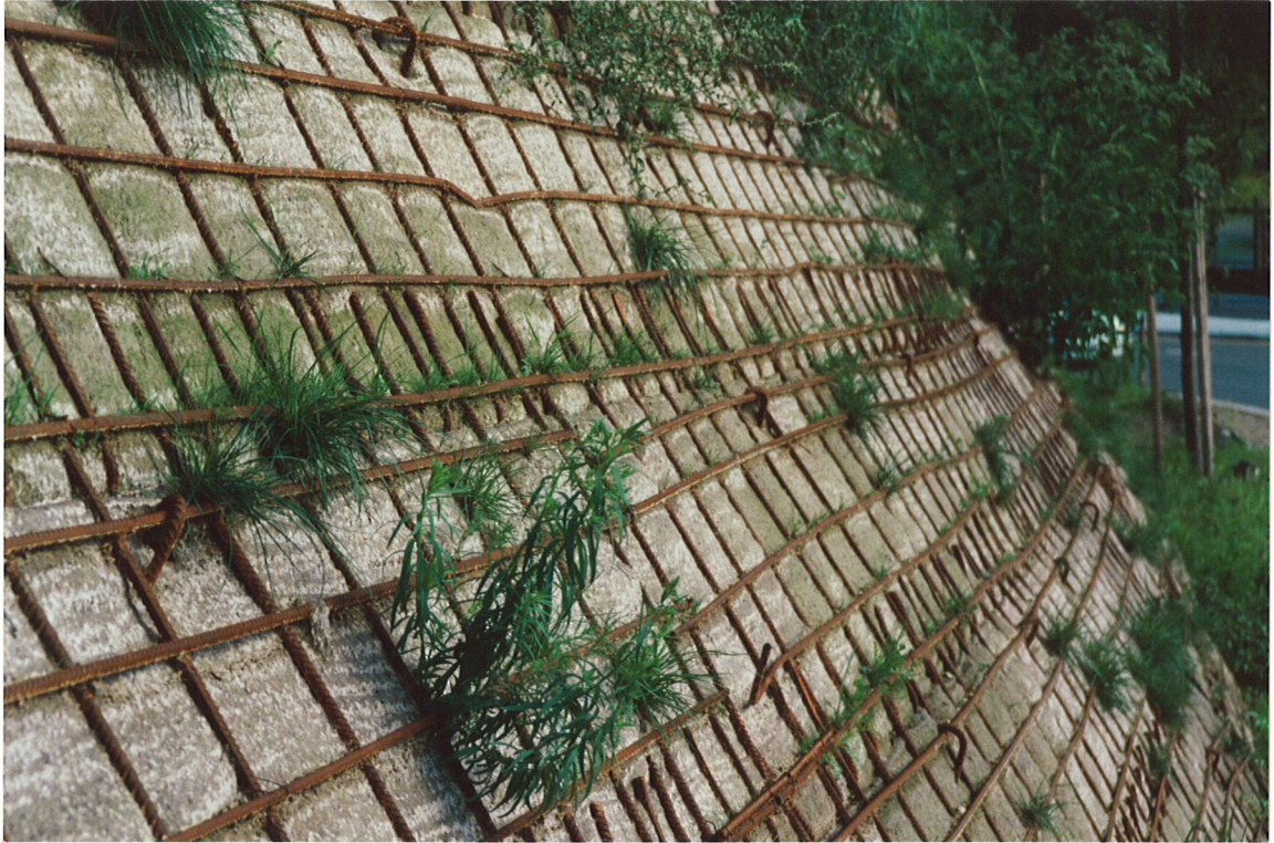
Fig. 13 Detail of the facing
