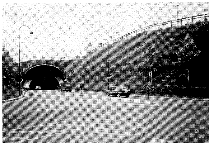
Fig. 3 Finished reinforced slope
