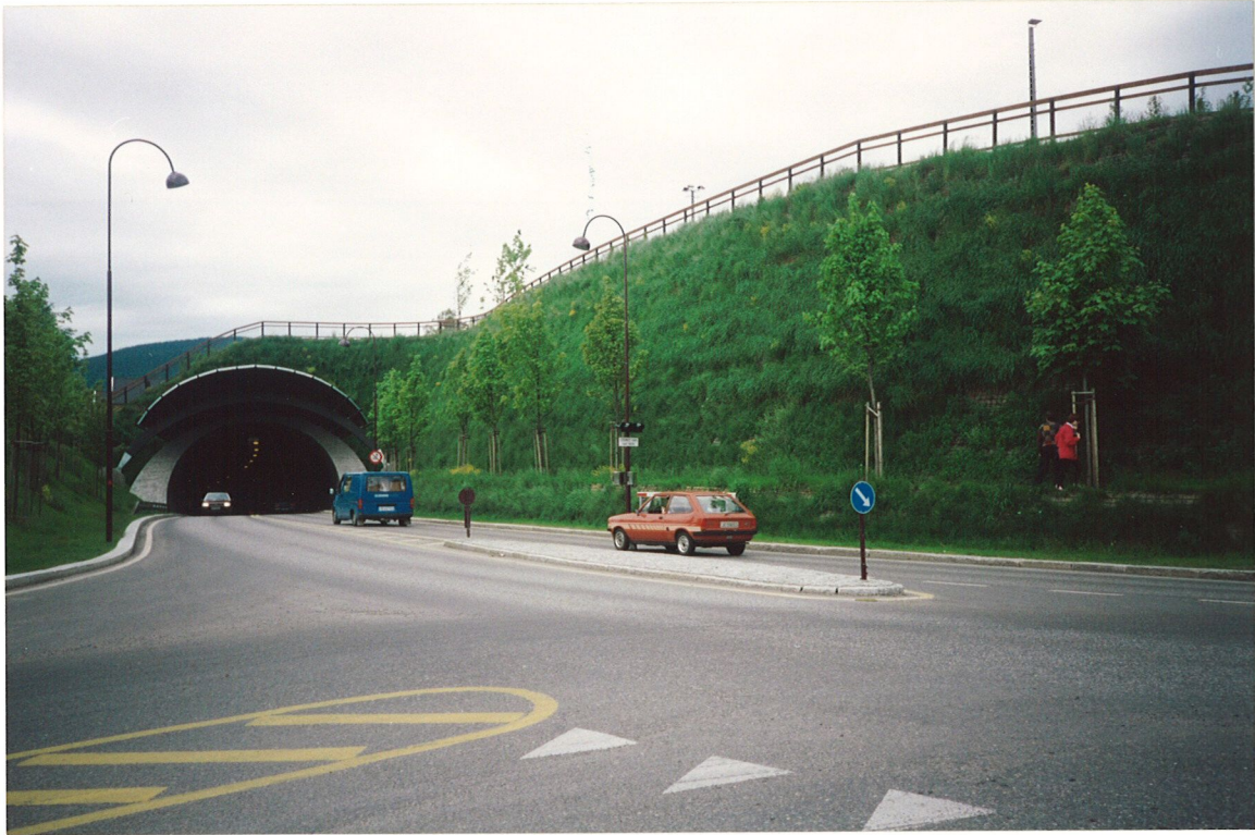
Fig. 15 Green slope finished
