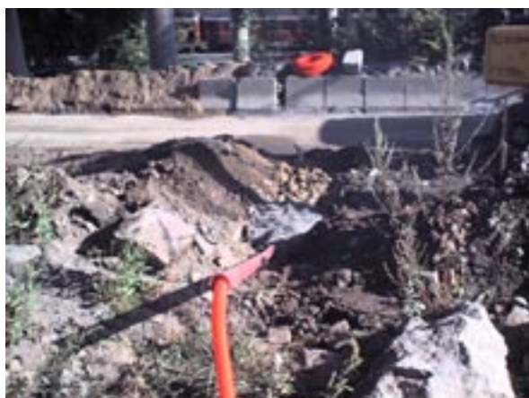
Figure 7: Monitoring long term deformations with tube settlement gauges.
