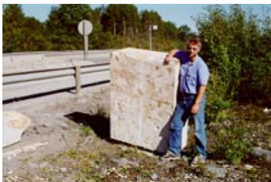
Figure 3: Excavation of a 24 years old EPS block from the first EPS embankment at Flom bridge.
