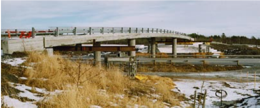
Figure 20: Temporary support of abutments at Hjelmungen.
