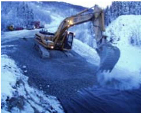
Figure 3: Placing of foamglass with excavator.
