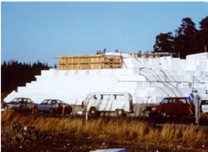
Figure 10: Construction of one abutment on the EPS embankments at Løkkeberg bridge.
