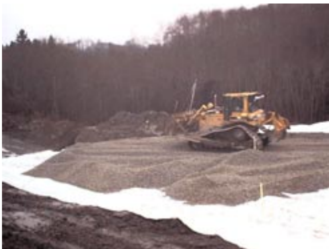
Figure 12: Distribution and compaction with dozer.
