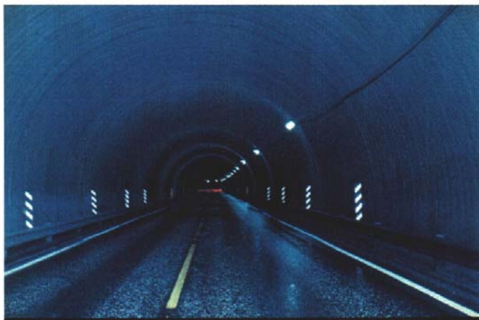
Figure 4: Water and frost protective panel made by corrugated aluminium sheets.
