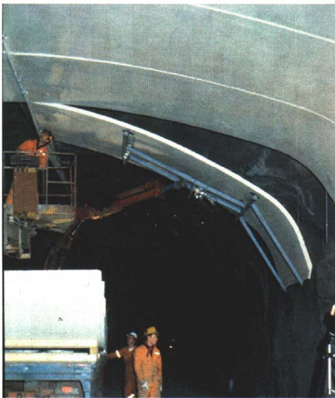
Figure 5: Installing the sandwich lining is efficient.
