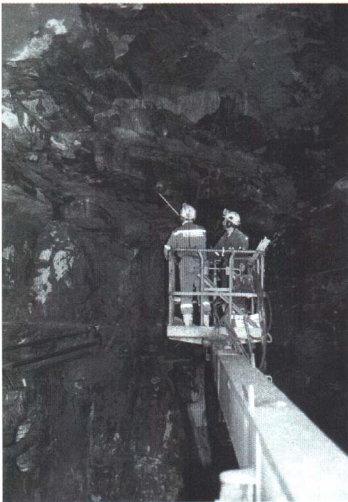
Figure 2: Rock bolting is extensively used for support.
