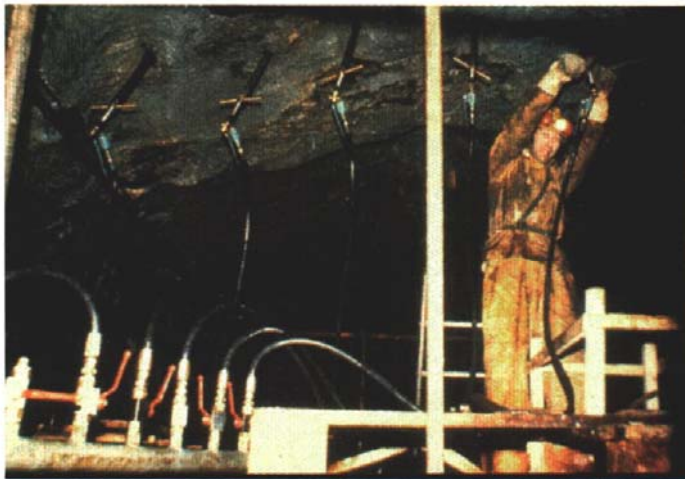
Figure 3: Grouting for water sealing by means of chemicals and high pressure.
