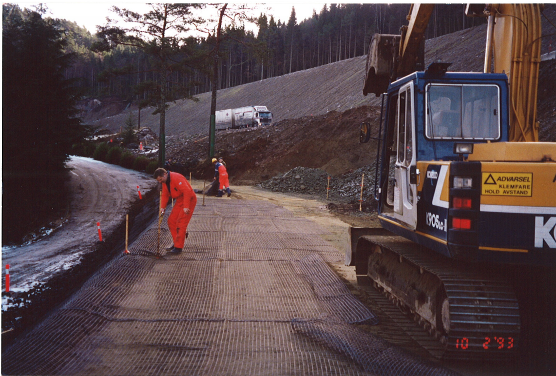
Fig. 7 Construction of 45 ° slope. Telegrid 55/30 used as reinforcement
