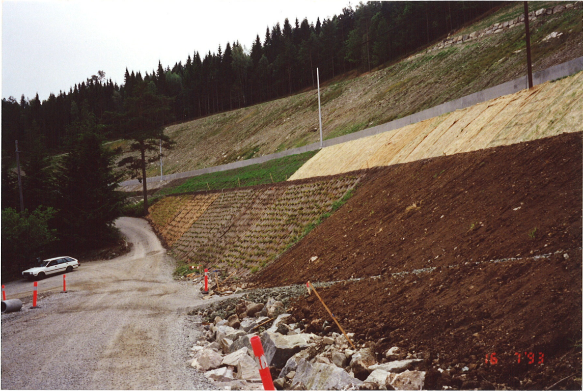
Fig. 8 Reinforced slope with test sections for different vegetation mats
