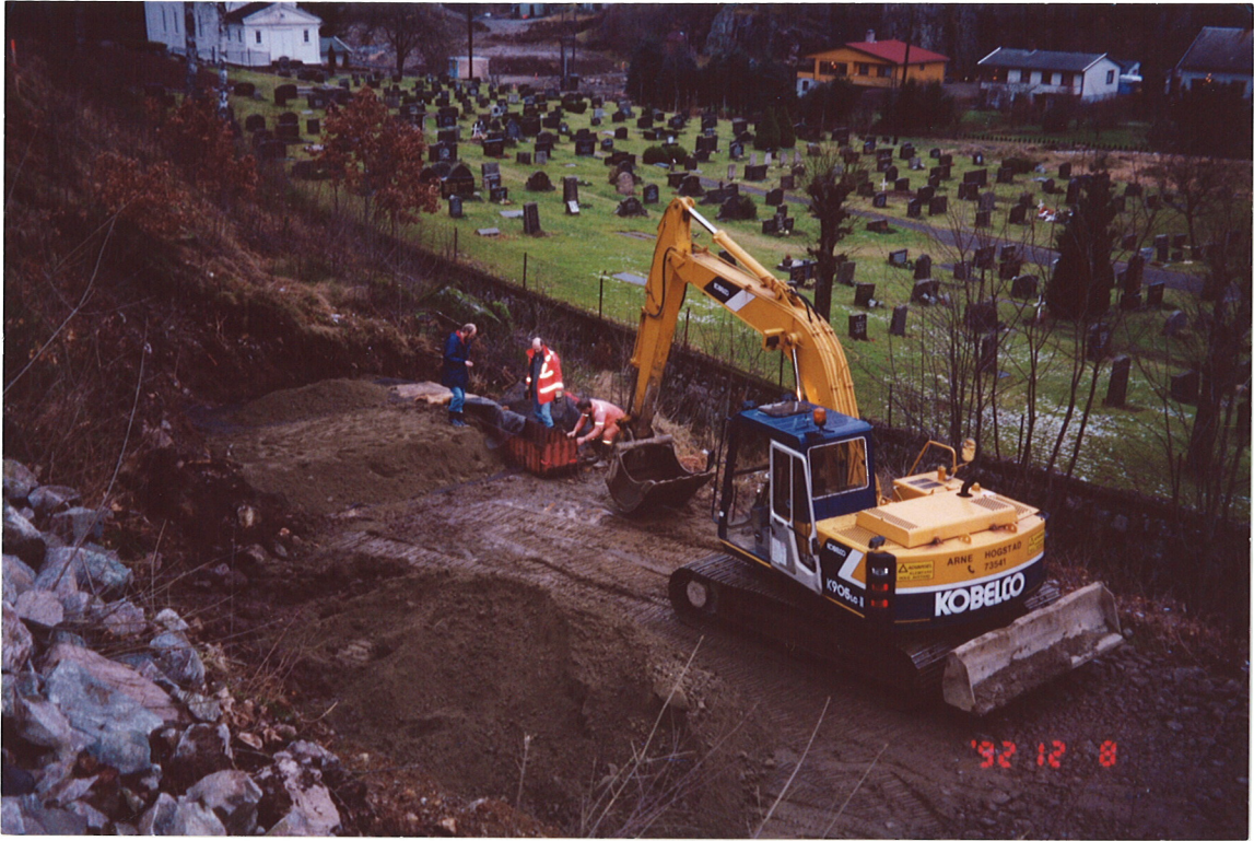
Fig 1 Construction of 60 ° reinforced slope, first layer
