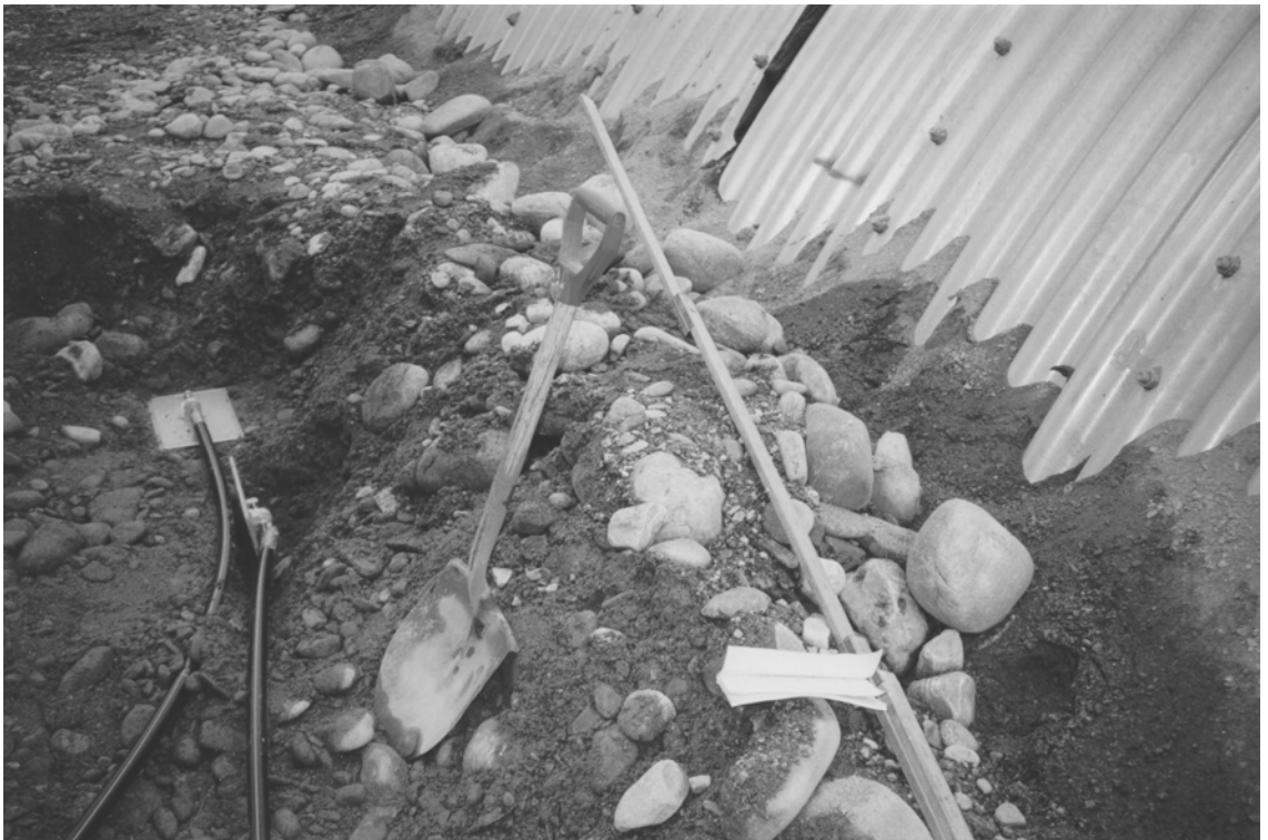
Figur 6 Jordtrykscellene log 2 under montering.
