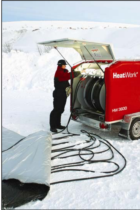
Figure 1. Hydronic-based defrosting system mounted on a trailer for in-situ thawing operations. After initial programming and start-up, the system is left on the site until the desired thaw depth is reached.
