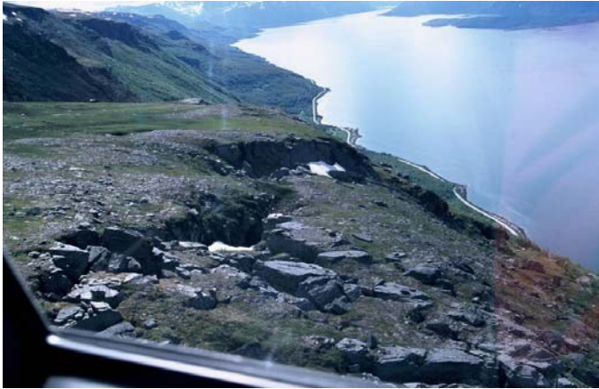
Figure 1. One of the major fractures at the Nordnes rockslide, experiencing active movements.
