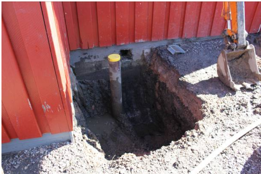
Figure 4: Pile installation
