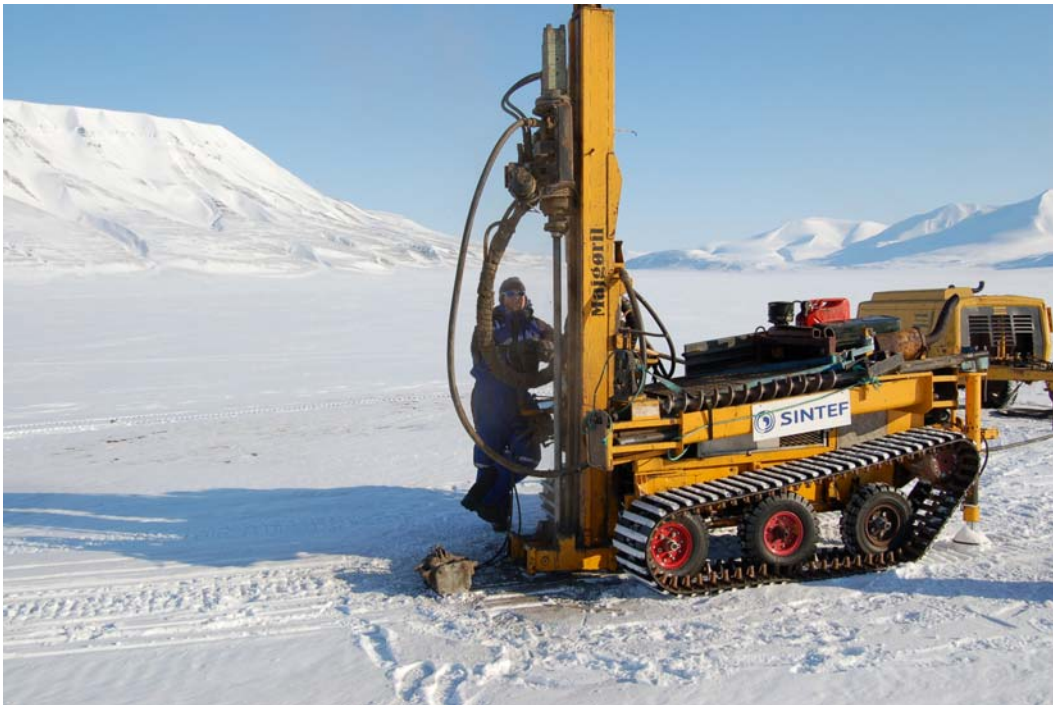
Fig 2. The SINTEF drill rig placed in Longyearbyen
