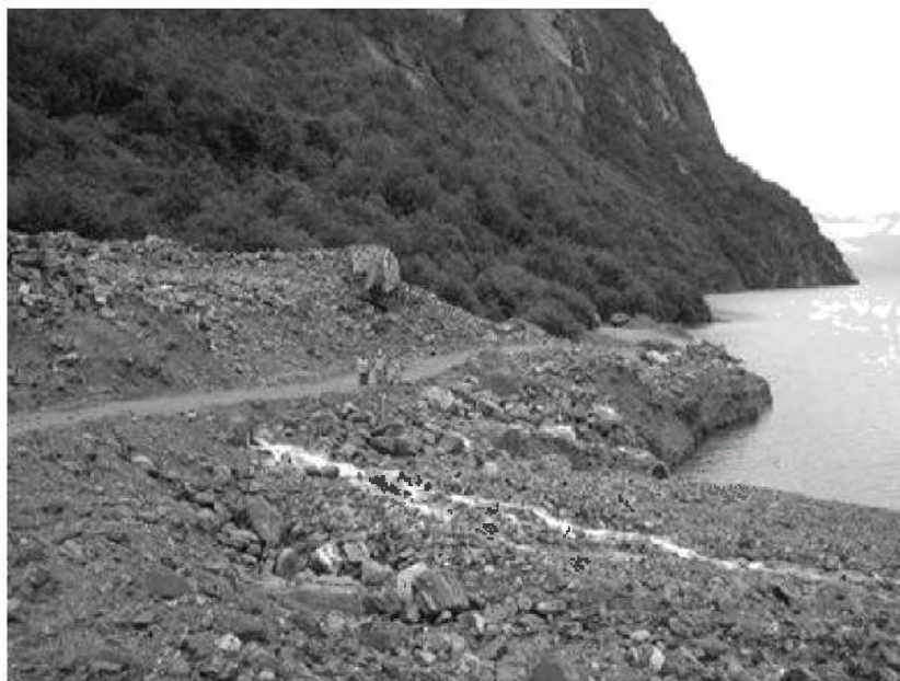
Figure 10: Debris flow as a consequence of a rain storm destroyed 300 m road. in Eikesdalen, West Norway (Photo: Jan Otto Larsen)
