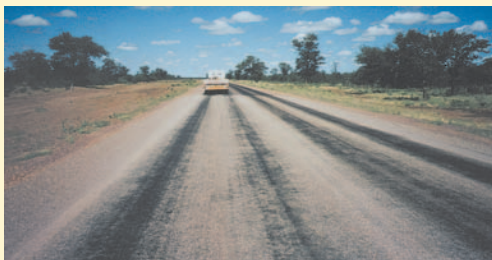
An Otta Seal will for the first few months after opening to traffic exhibit a rich bitumen appearance, which initially appears non-uniform and inferior compared to the conventional Chip Seal. (Botswana).
