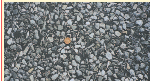
Close-up of the Otta Seal surfacing. (Norway).
