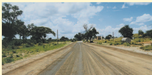
Correct aggregate application rate. (Botswana).
