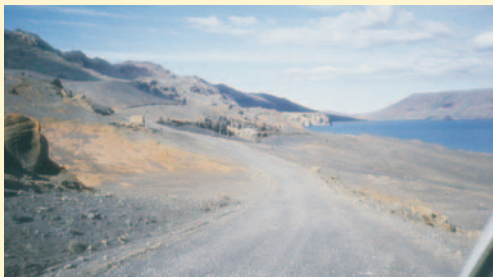
A newly laid Otta Seal using crushed basaltic gravel. (Iceland).
