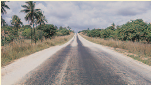
A section where coral stone was used as Otta Seal aggregate. The first section has been in service for some months and the aggregate has "bed down" making an appealing and uniform appearance. The second section has newly been constructed and the coral aggregate still need some time to "bed down". After more than 14 years in service these sections are performing excellently. (Kenya).
