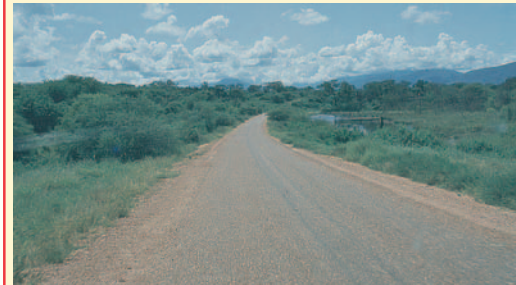
Turkana road, about 20 km north of Marich Pass. Screened quartzitic gravel were used as aggregate for the Otta Seal. After a number of years in service the performance was good. (Kenya).
