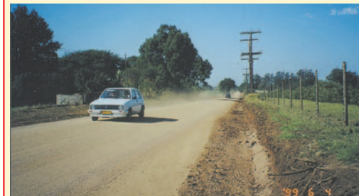
Unsealed roads very often provide an unsatisfactory driving comfort and associated high maintenance and operational costs. Dust pollution is also a problem in urban areas. (South Africa).
