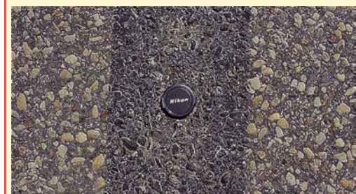
Otta Seal with sand cover seal, where the dense matrix is further enhanced. (Botswana).
