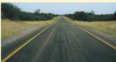
After some months in service the Otta Seal "beds down" and provide an uniform appearance. (Botswana).
