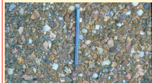
Close-up of the graded aggregate used in the Otta Seal. Note the dense matrix and interlocking.
