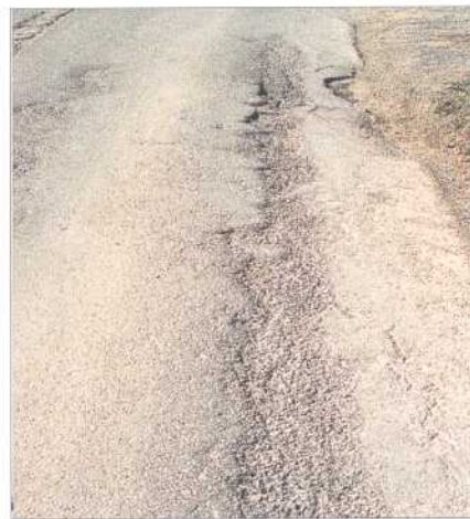
Ujevn overflate,, Alvorlighetsgrad H
