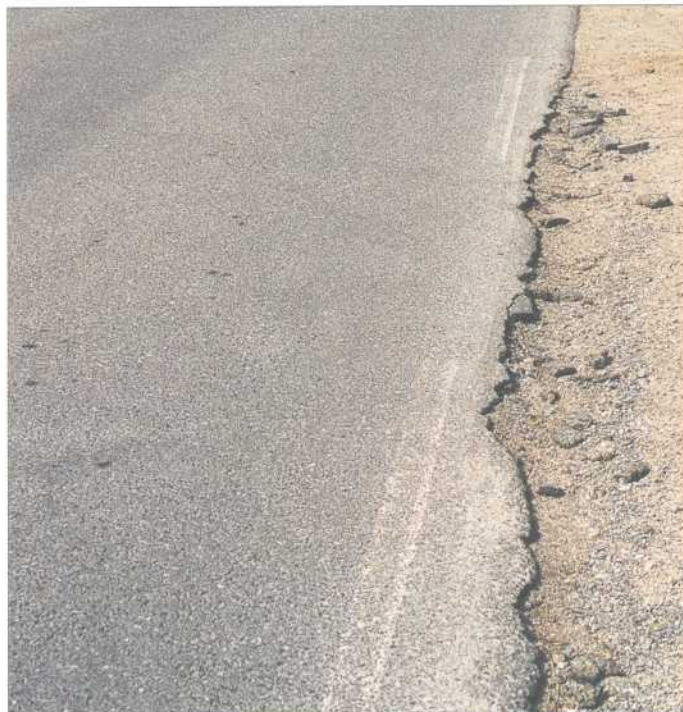
Lurvekant, Alvorlighetsgrad M
